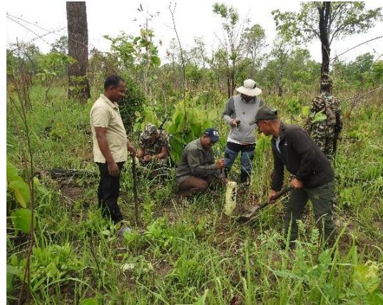
Figure 4: Staff installing a concrete pillar
