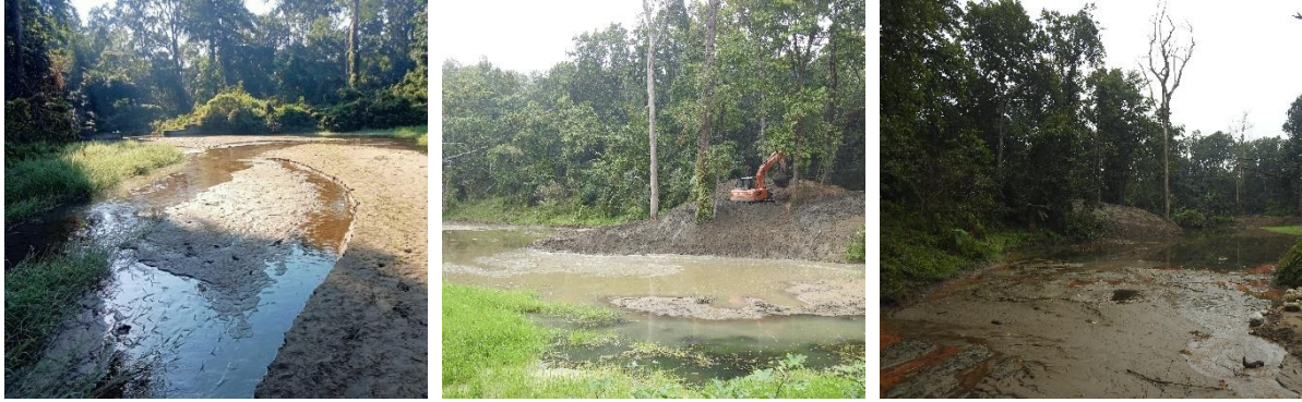
Figure 26: Photos of Kalidaha lake siltation (left), silt removal (middle), and after (right)
