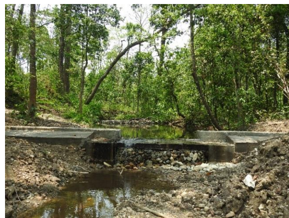
After construction of second checkdam
