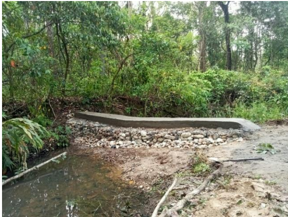
After construction of first checkdam
