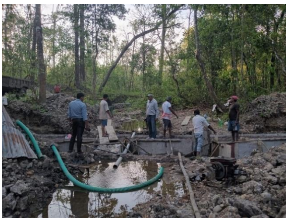
Ongoing construction of second checkdam
