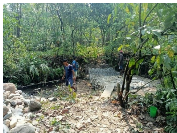
Ongoing construction of the first checkdam
