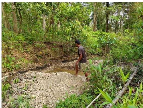
First checkdam construction site before construction
