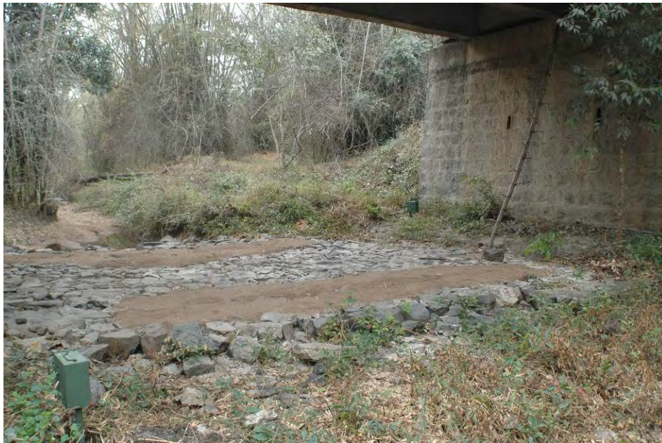
Camera traps were placed under culverts with varied structural dimensions to assess their usage by wildlife to cross the highway - © Sanjay Gubbi
