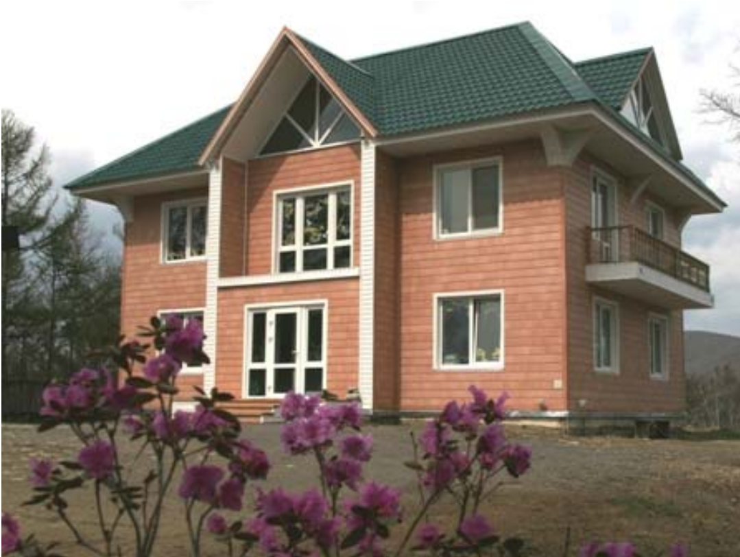
Photo 1. The Sikhote-Alin Research Center, Spring 2008. ©WCS
